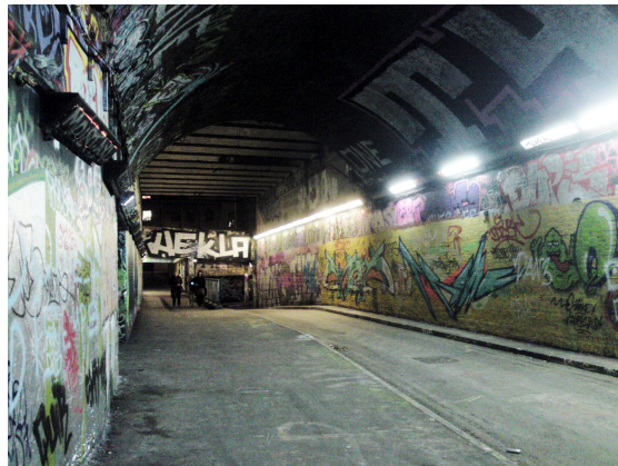
Figure 1: One of the many graffiti walls scattered across the city
